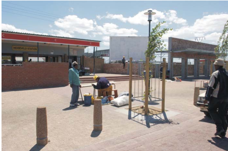
HEIDEVELD STATION - GUGULETU SIDE - BEFORE UPGRADE
